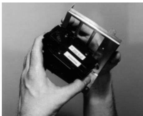
Figure 2. Installation of Circuit Breakers
